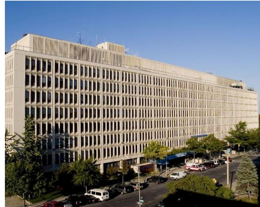
In addition to interior renovation, the recommended Current Hospital Reinvestment project includes exterior envelope upgrades. Existing windows allow excessive air and moisture into the building, which can compromise infection control and disrupt patient recovery. External envelope upgrades will address these issues and replace the existing windows with properly sealed units.
